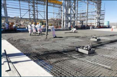
Heavy, labor-intensive traditional reinforcement
